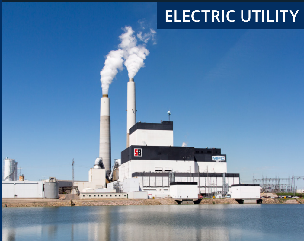
Coal-Fired Power Plant
